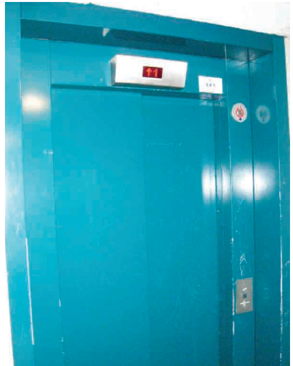
Schachtoegang in conditie 2
