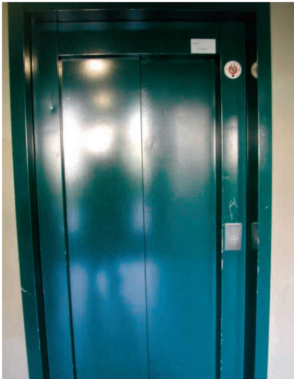
Schachtoegang in conditie 2
