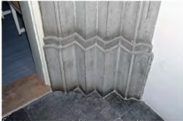
TK-A-254 Details hardstenen bekleding.
