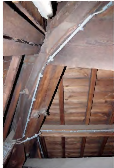
TK-A-239 Grenenholten dakbeschoot.
