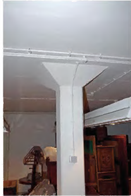
TK-A-250 Detail paddenstoelkolom.
