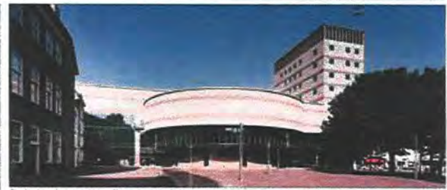
The canopy and green steps seen. The workings of the Parliament are brought into contact with the street level.
